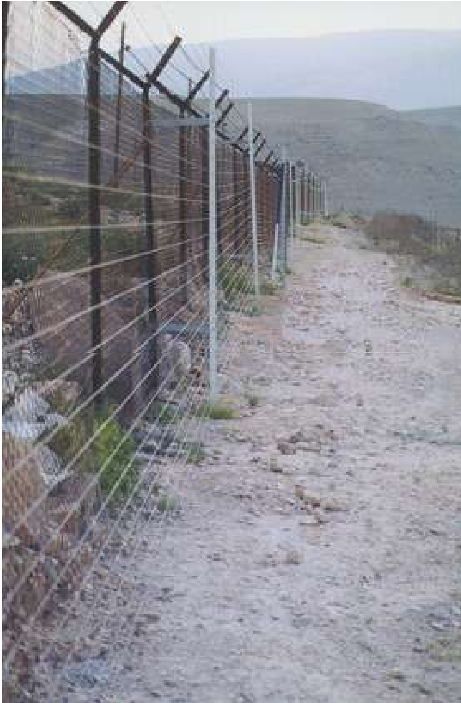
Installation of electric fence wires on an existing fence
