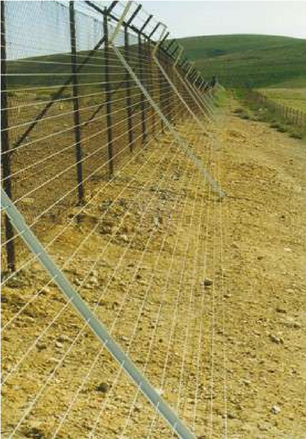
Installation of electric fence wires on an existing fence
